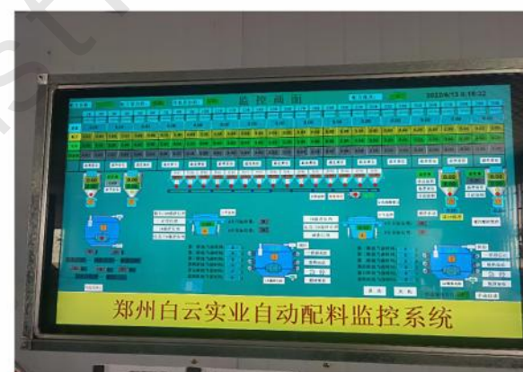
配料监控系统 Ingredient monitoring system
